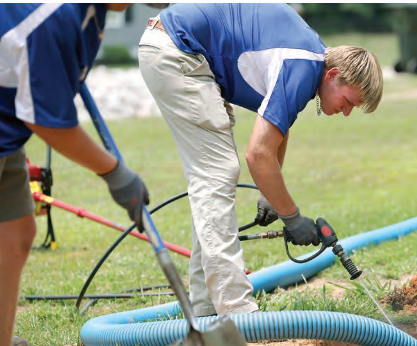
▲ Hunter Creech washes down a septic tank during a service call. The company's vacuum truck is equipped with an onboard jetter/washdown system from Pumptec.
