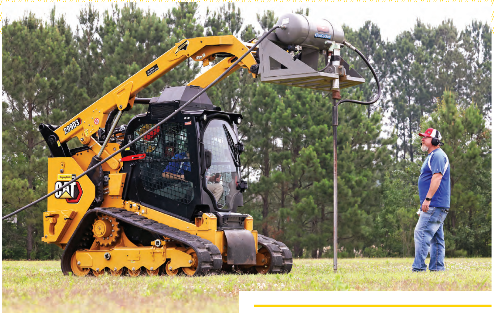
▲ Hunter and Stacy Creech use their EarthBuster drainfield rejuvenation equipment from K&P Enterprises. The attachment is mounted to a Cat skid-steer in the field.
