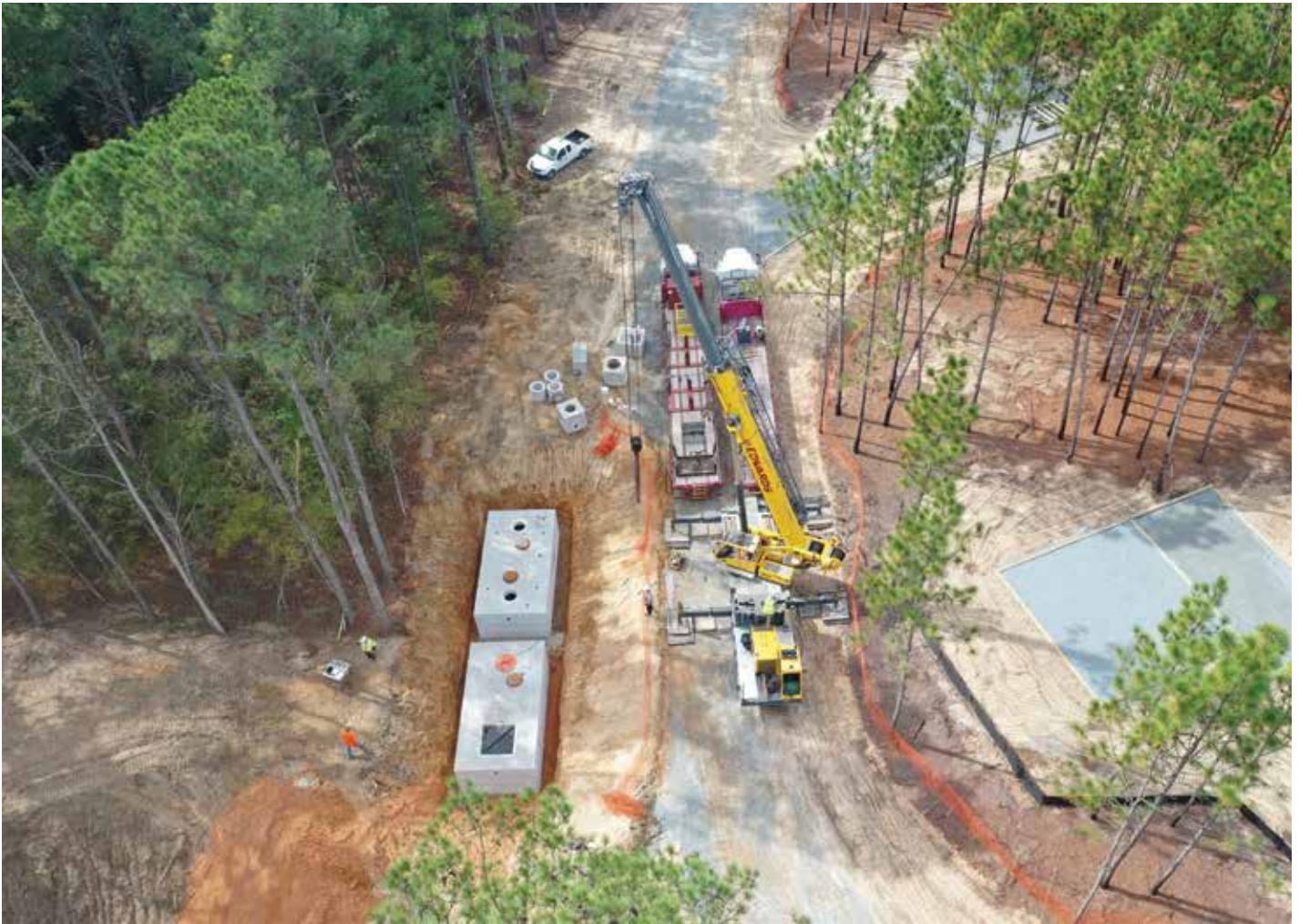
Each tank consisted of three sections, with the top and bottom sections weighing 21,000 pounds a piece and the middle 14,000 pounds.
