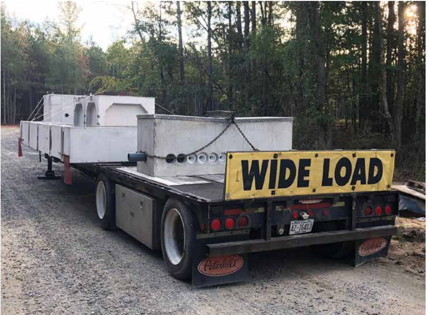
The project site was on a narrow ranger road and more than two hours from the Shoaf Precast plant, requiring careful planning for transportation.
